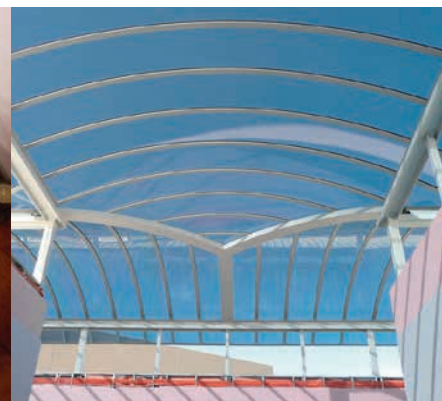
Applications of PC or PMMA flat sheets in the construction sector such as skylights, roofs, and greenhouses.
